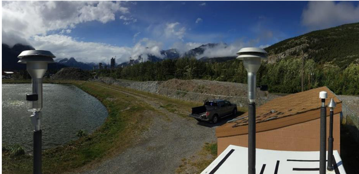
Figure 3-1 Inlets on the top of WSP's Lagoon Station
