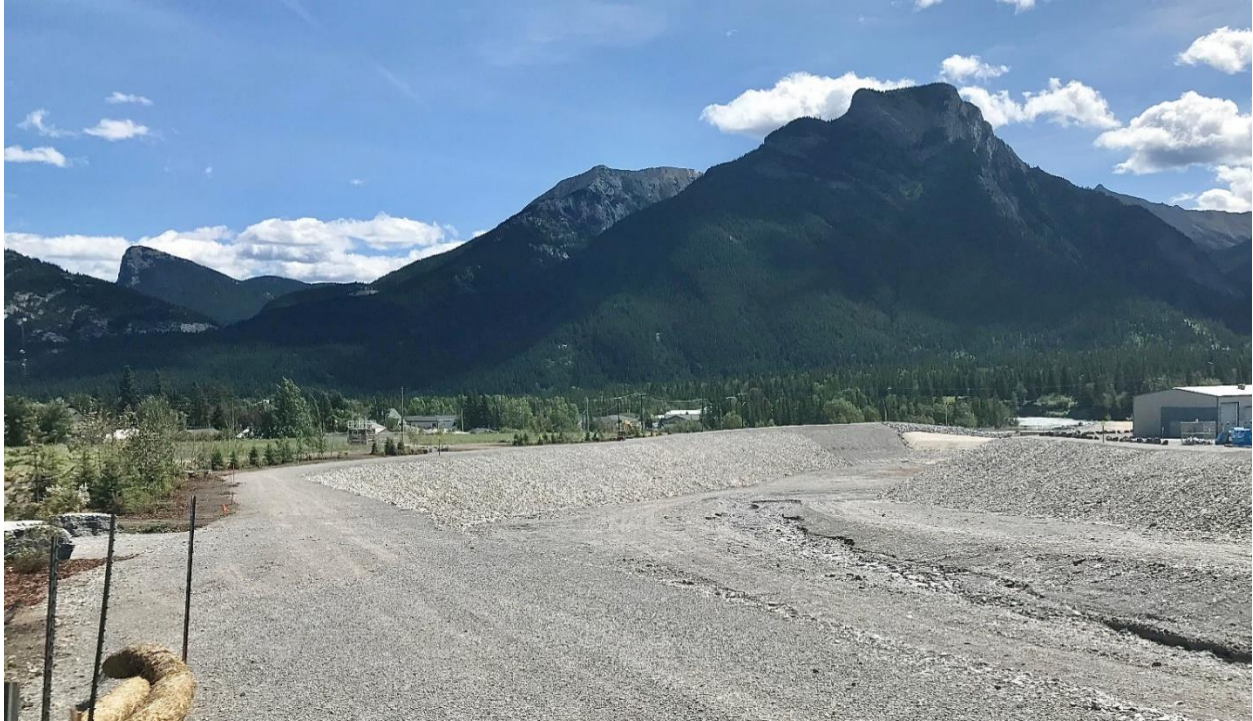
Figure 1-2 Photo of Completed Flood Mitigation Work at Exshaw Creek
