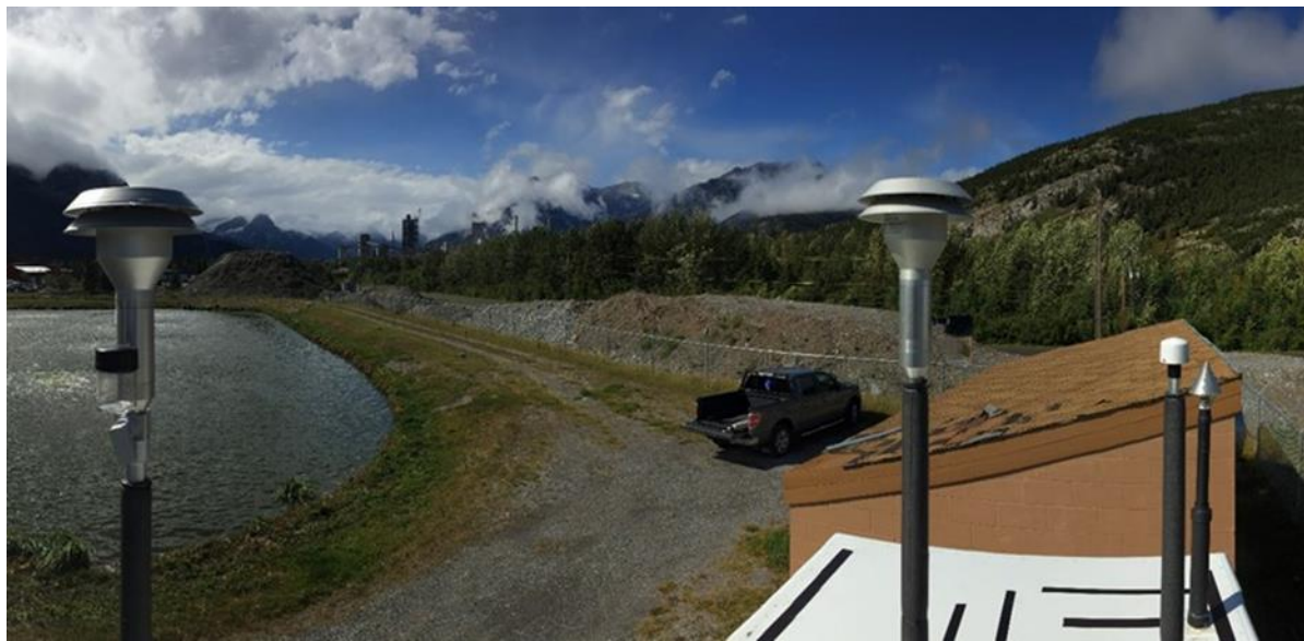
Figure 3-1 Inlets on the top of WSP’s Lagoon monitor
