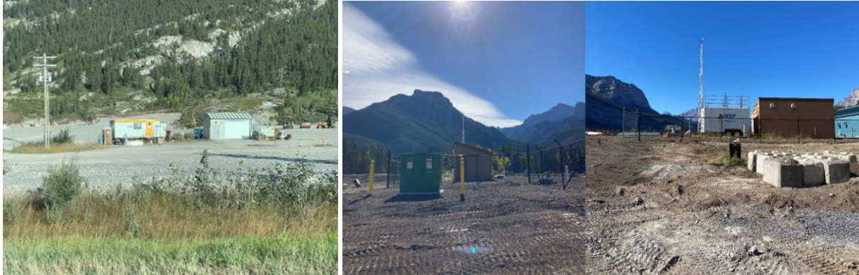
Figure 1-3 Photo of Residential Development (Left) and Construction of an Additional Lagoon Pond in East Exshaw (Right)
